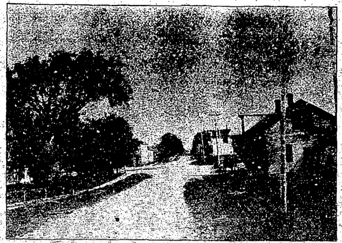
This picture was taken from near the Baptist church and is looking north from spot. G. E. Gough's store is shown on the corner opposite the post office. Wright, while across the street further north a portion of Charles Green's hotel and H. H. Jones store is seen. The photo was taken by "Pat" Quinn.
