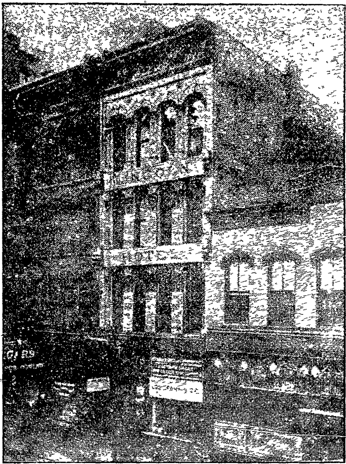
The Lincoln Hotel, Chicago, where the Northville people had such a narrow escape from burning to death. They occupied the top room on the right.
