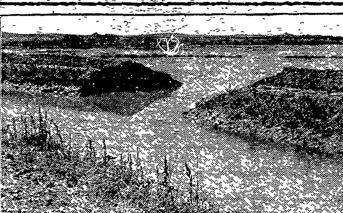
BREAK IN DITCH CAUSED BY GROUND SQUIRRELS.
