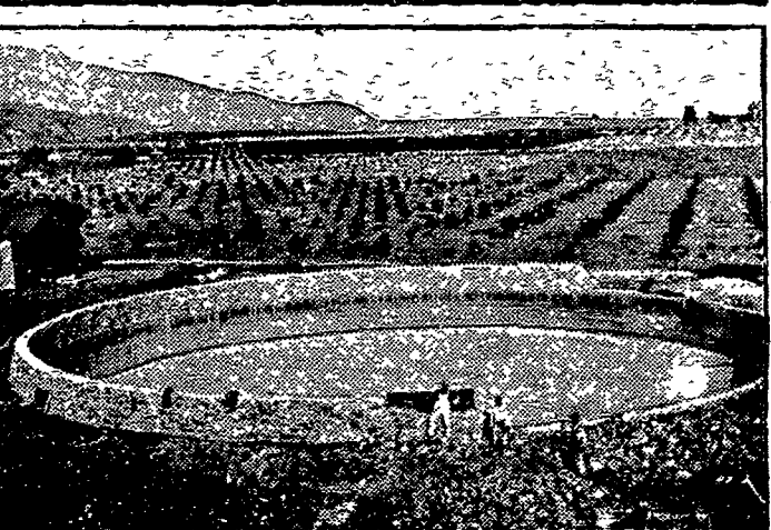
BUILDING COBBLESTONE WALL OF RESERVOIR.
