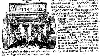
will handle manure—fresh of will namine manure—iresit or stored—easily, economically and efficiently. A chain conveyor carries the manure to two cylinders, revolving one over the other, where it is thoroughly fined and pulverized. Then, swiftly revolving steel paddles distribute this fine manure a write wider than the
