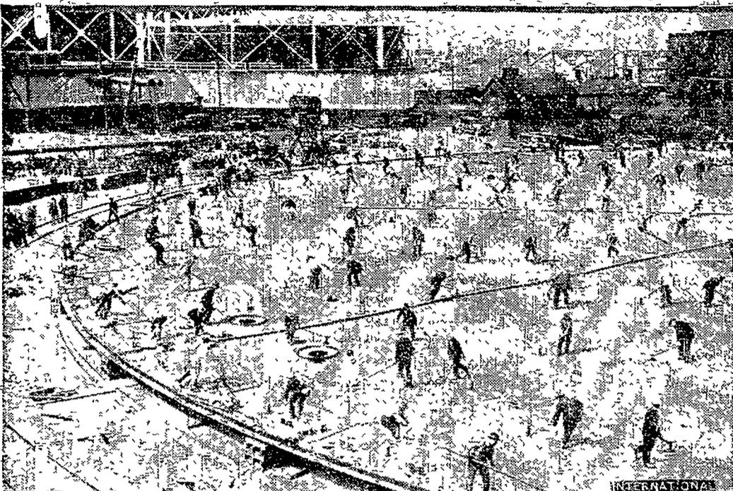
More than one hundred workmen lowering the large base of a 10,000,000-cubic-foot gas tank for the Pacific Gas & Electric company into position in San Francisco. The tank will be 28 feet high and 276 feet in diameter. It will be of the telescopic type, having five collapsible sections.
