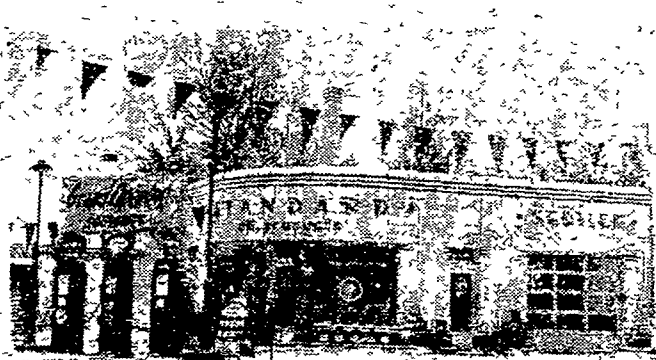
The newly constructed Bailey Standard Oil Service station will hold its formal opening Friday, Aug. 2. To celebrate the event the management is offering gift awards and special services to persons who visit the new plant.
