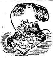
OF SPEECH - Western Electric Company, the Bell System's manufacturing division, uses materials from all over the world to make your telephone. The newest-type telephone has 433 parts and is made of 48 different materials. Among them are iron, steel, nickel, copper. un, lead, zinc, aluminum, chromium, magnesium, gold silver, platinum, coal, cotton, silk, paper, "ubber, wax, shellae, asphalt, clay, tale, mica, leather, wood.
