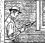
the leaks. You should force the compound in around the window frames on the butside of the
