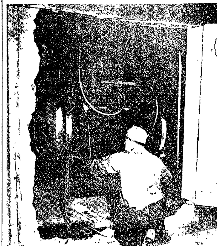
The Kluge press comes down the elevator shaft of the new building at the corner of Main and Center streets. The press was taken into the building via the loading dock on the Main street side, suspended by two block and tackle rigs, and lowered down the shaft. The 2,000 pound press, as most other equipment in the shop, was too heavy for the elevator.
