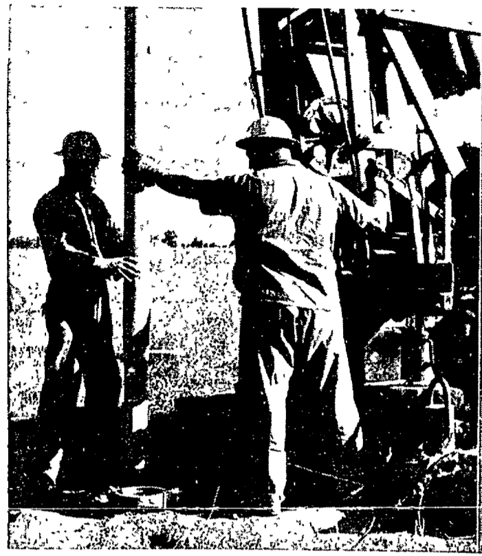
DRILLING A TEST WELL for water on the proposed Wixom Rd. site of the Lincoln headquarters and assembly plant has been keeping drilling crews busy from early morning until late at night. The crews, working for the Layne Northern Co. of Lansing, were running a preliminary test of water conditions in the area to determine if the potential output would be sufficient to supply both the factory and surrounding homes. In the above photo, James Fields, left, and Edward Mossman lower the drill into the partially drilled hole.
