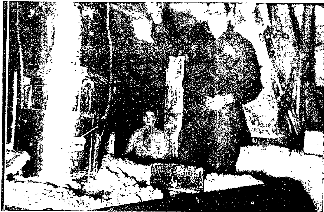
The ground-up apples fall through the vertical metal chute onto racks which are covered with heavy cloths. Ten of these racks, stacked one upon another, are called a "cheese". The cheese goes under a belt-driven screw press which extracts the cider.
