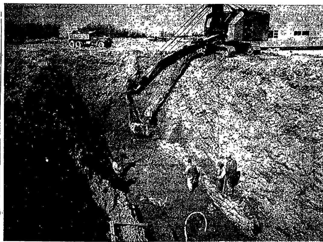
WORK IS PROCEEDING according to schedule at the site of the new Lincoln plant, according to company officials. Excavations are being made (above) for a sewage disposal system to carry off waste from the painting operations in the new assembly plant. In the upper left is the C&O railroad spur entering the plant from the north. The long house trailer behind the power shovel is one of many such trailers on the site housing construction company offices.
