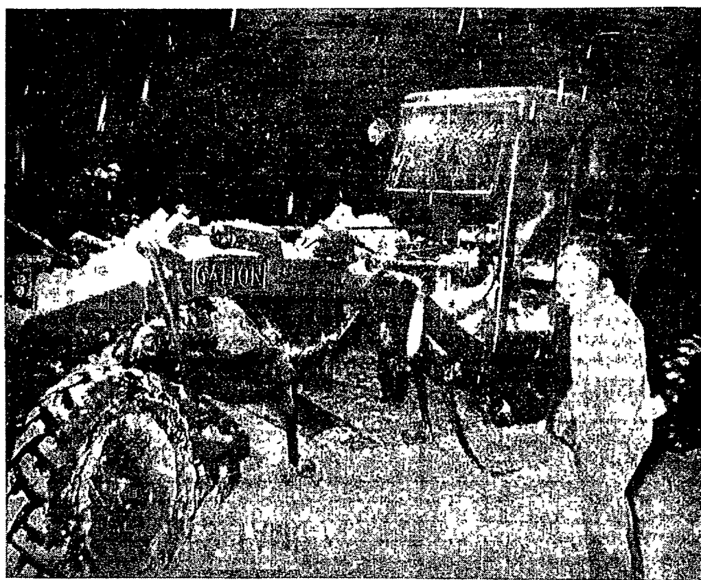
LOOKING something like a wet dog about to shake itself, Northville's road grader was pulled from its icy resting spot in the mill pond Saturday night. Members of the G. F. Taft construction firm, city employees and a huge wench combined to pull the grader out. A tow line, attached to the grader by Driver Bud Hartner before it sank was credited with making the chore possible. Extreme cold made the operation more difficult. Workers got relief in the form of hot coffee supplied by Paul's Sweet Shop.
