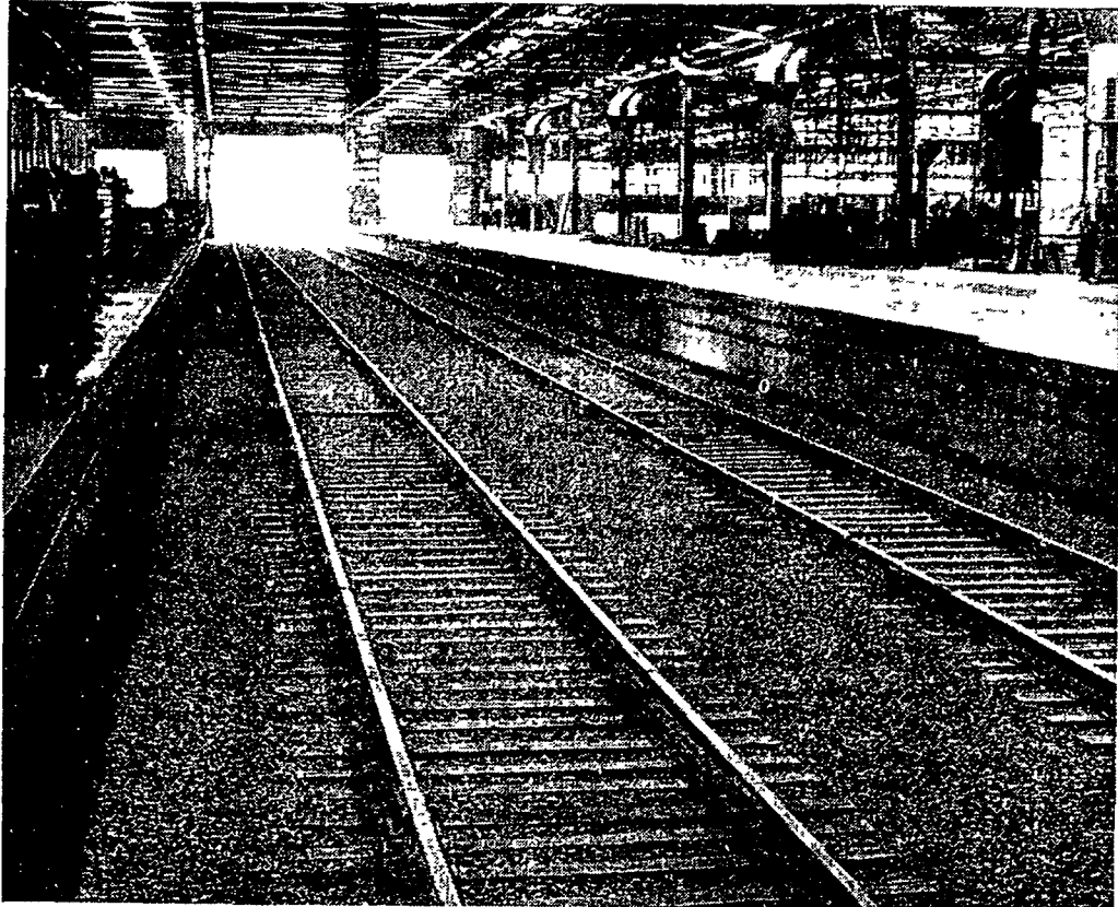
SOME 34 RAILROAD CARS can be accommodated simultaneously in the new Lincoln plant where 1,080 tons of materials will be unloaded daily. There are also facilities for handling 24 trucks. The tracks are located inside the plant in such manner that freight cars can enter or leave either end of the manufacturing building.
