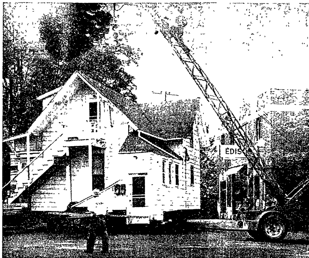
STARTING out on its trip to a new location, the house makes a careful turn at Center and Dunlap as workman (top of picture) watches power line clearance.
