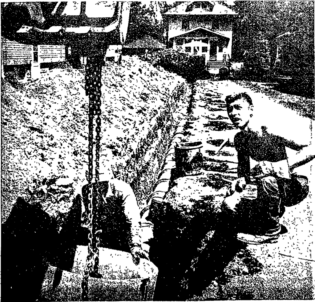
TRENCHING for storm sewers on Wing, First and Fairbrook streets was well underway this week. The work began the first of June and will be completed by August 31. Curbs and gutters will be installed when storm sewers are completed. The above picture was taken on Wing street.
