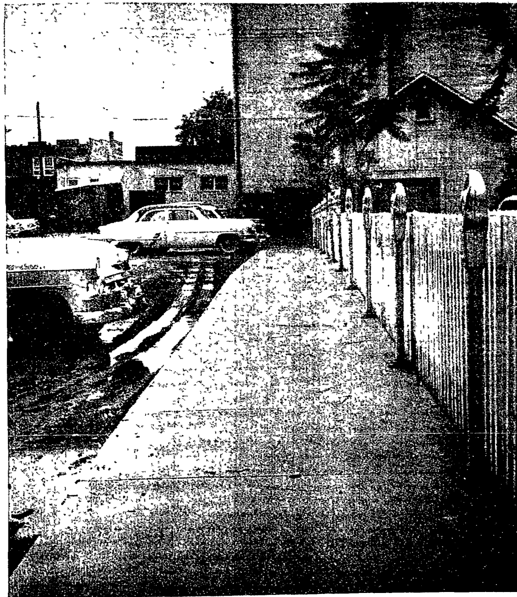
PARKING METERS and new walks have been installed to accommodate 25 cars at the city's new Dunlap street lot directly behind Main street stores. City councilmen have decided that parkers will enter from Dunlap and exit through an alley leading to Hutton street. The walks allow shoppers convenient entrance to stores in the area and also protect the meters from being bumped by parkers. The meters are set for nickels, dimes and quarters allowing 2-hour, 4-hour and 10-hour parking.
