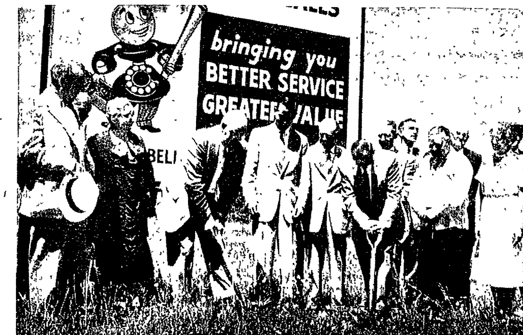
DIGGING FOR DIALS! Northville's Mayor Claude Ely and Frazer Staman, Novi township supervisor, turned the first shovels for the new $1,425,000 Michigan Bell Telephone company dial exchange building in Northville Monday. The exchange, which will serve the complete area, will be in operation July, 1958. City, township and telephone company officials watch as Ely and Staman sink their bronze-plated shovels.
