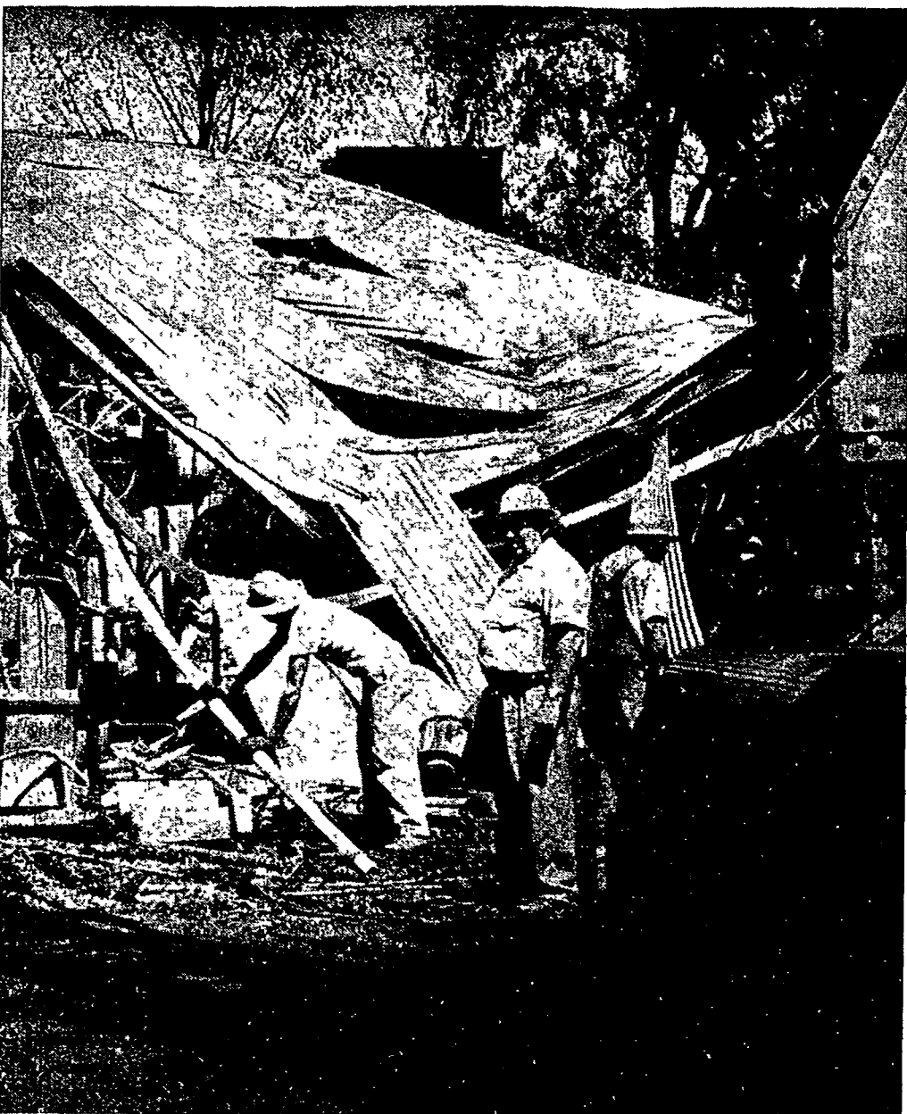
DOWN IT COMES — Wreckers begin demolishing what is left of the Allied Products division in Northville. Shown here is one of the most severely damaged areas, where the fire was so intense that the quenest shell buckled and collapsed like a deflated balloon. Operations were halted this week while insurance investigators completed their survey.
