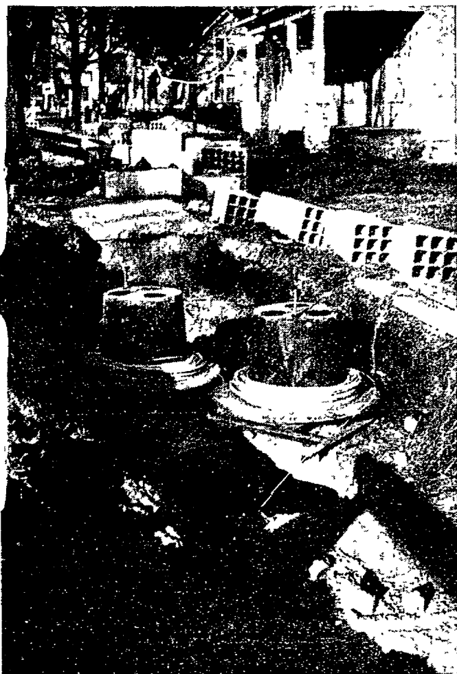
SIDEWALKS UPROOTED — Those neat stacks of tile tubing that lined North Center street began to disappear last week. They're going underground — beneath the sidewalks — to carry cable to the new Michigan Bell Telephone exchange building. Most of the walk along the east side of the street has been removed from Rayson northward to Baseline. Dial service is scheduled for the Northville-Nowi area in July.
