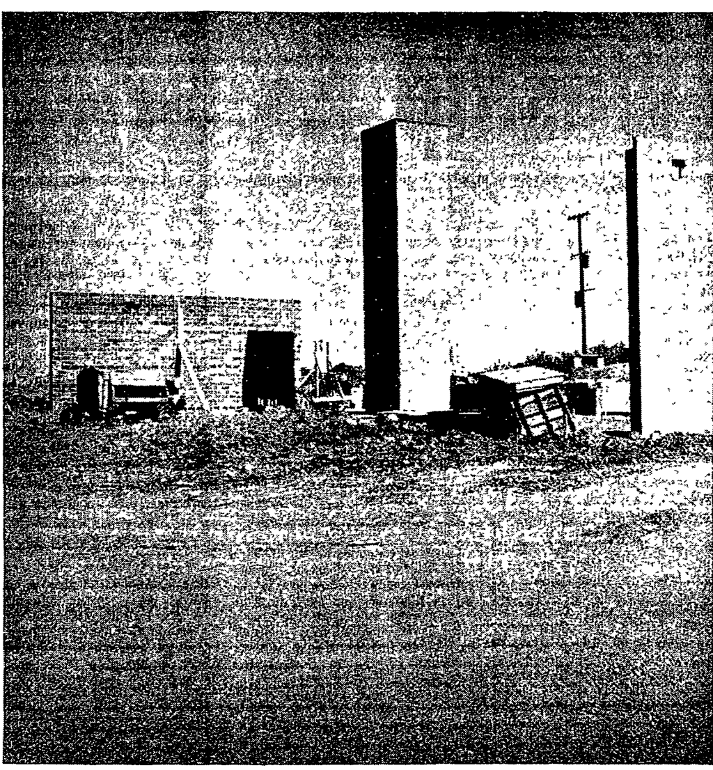
IT'S A START - Northville's new high school began taking shape last week with the erection of walls for the power plant wing. Also in the wing will be driver training headquarters and manual training shops. Work is coming along well on other buildings at the North Center street site.
