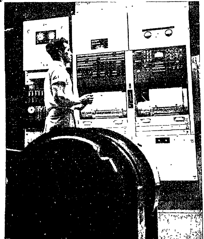
DOUBLE CHECK—Edward Simetz, of Livonia, a Western Electric installer, takes readings at the new Northville exchange building's power control board to make sure the equipment is ready for the conversion to dial service. Generator is in foreground.
