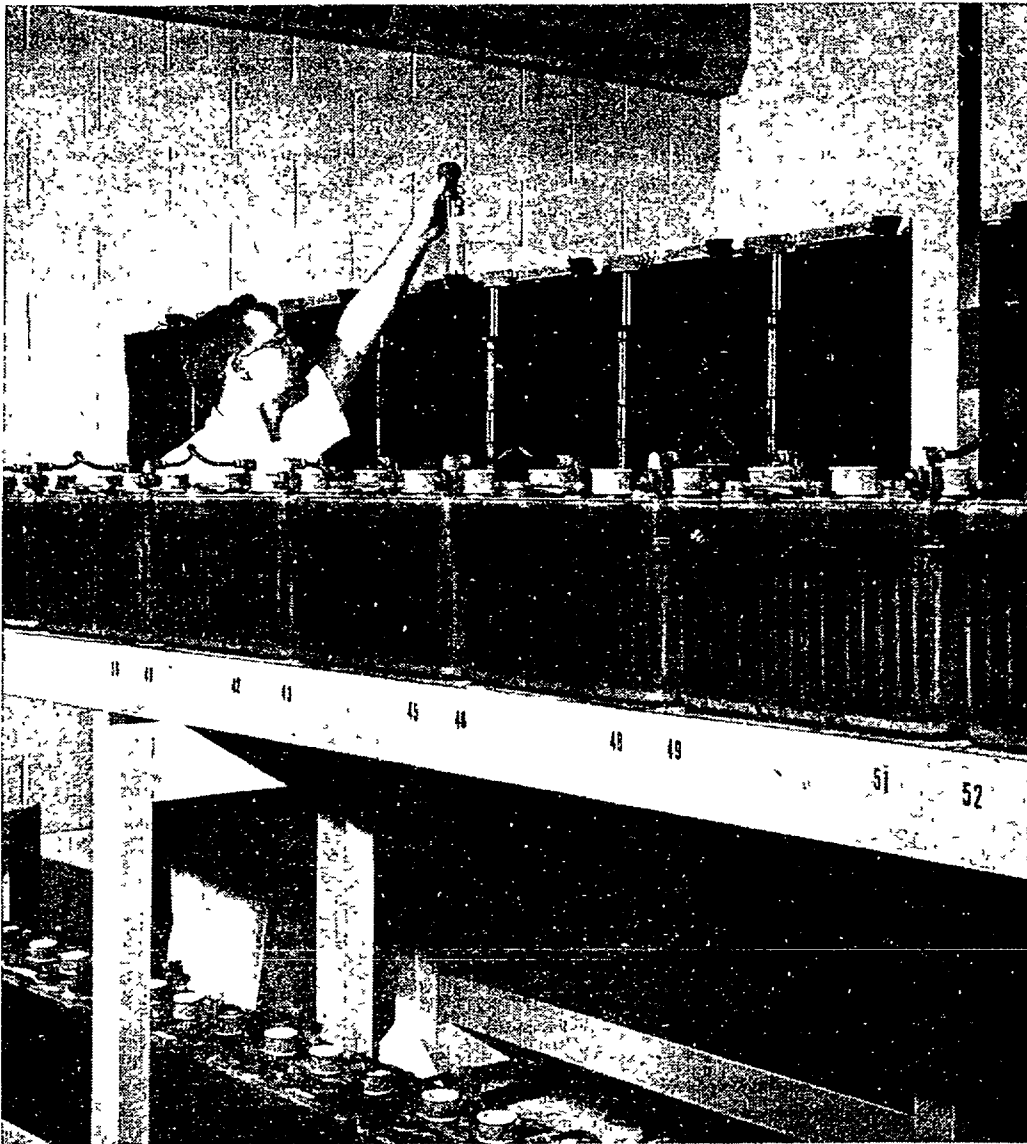
Richard Scruggs of Dexter, a switchman, checks batteries in the power room of the new Northville exchange building. The huge batteries will supply electrical current for the dial system.
