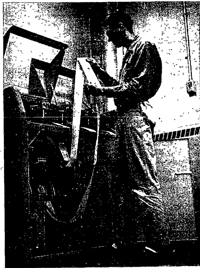
AUTOMATIC MESSAGE accounting equipment goes into operation along with Northville's new dial system. Here, Chester Sandeck, a Western Electric installer, reads the tape which records dialing information such as the calling telephone number, the party dialed, and length of call.
