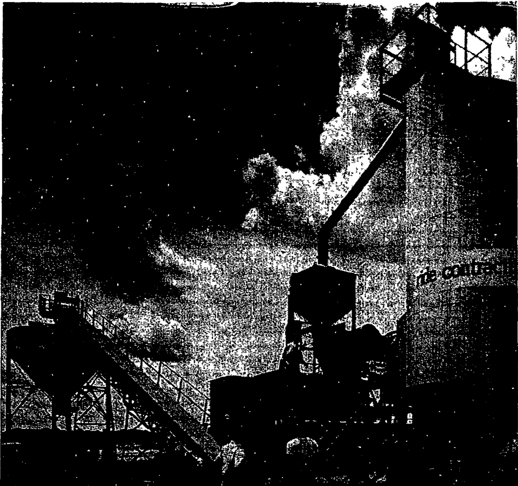
HOME OF POZ-O-PAC—Ride Contracting, Inc., recently installed this $102,000 plant on West Seven Mile in Northville, where it will produce "Poz-O-Pac", a base construction material for highways and airports. The plant, covering 40,000 square feet, can produce 400 tons of the material an hour. Poz-O-Pac forms in- to a concrete-like base that is impervious to weathering and traffic. General offices are in Oak Park.
