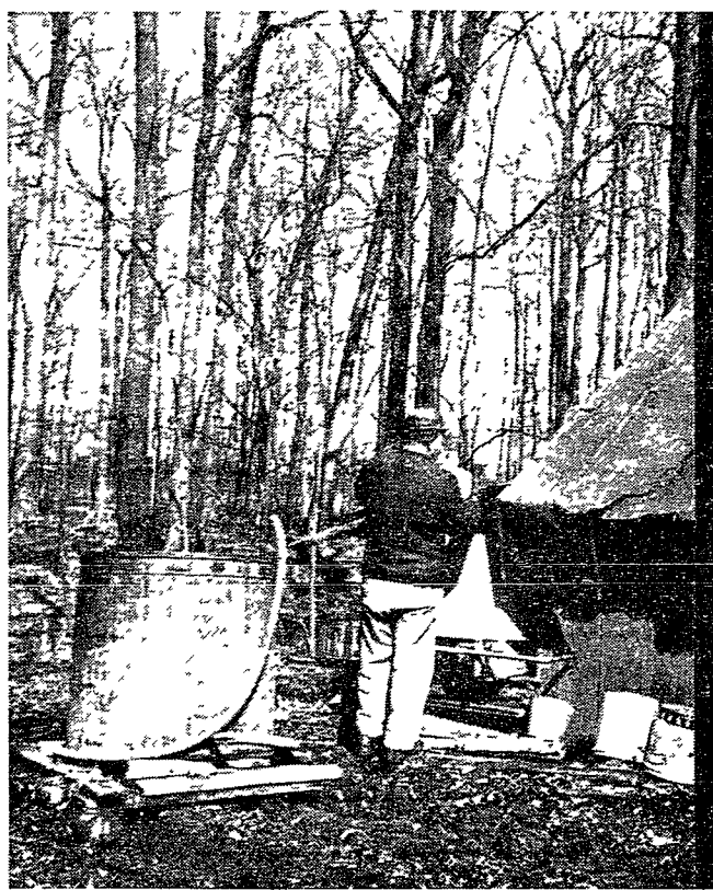
INTO THE STORAGE TANK — After the sap is gathered from the tree pails it is poured into the tanks outside the hut. From there it runs into the evaporating pans inside.
