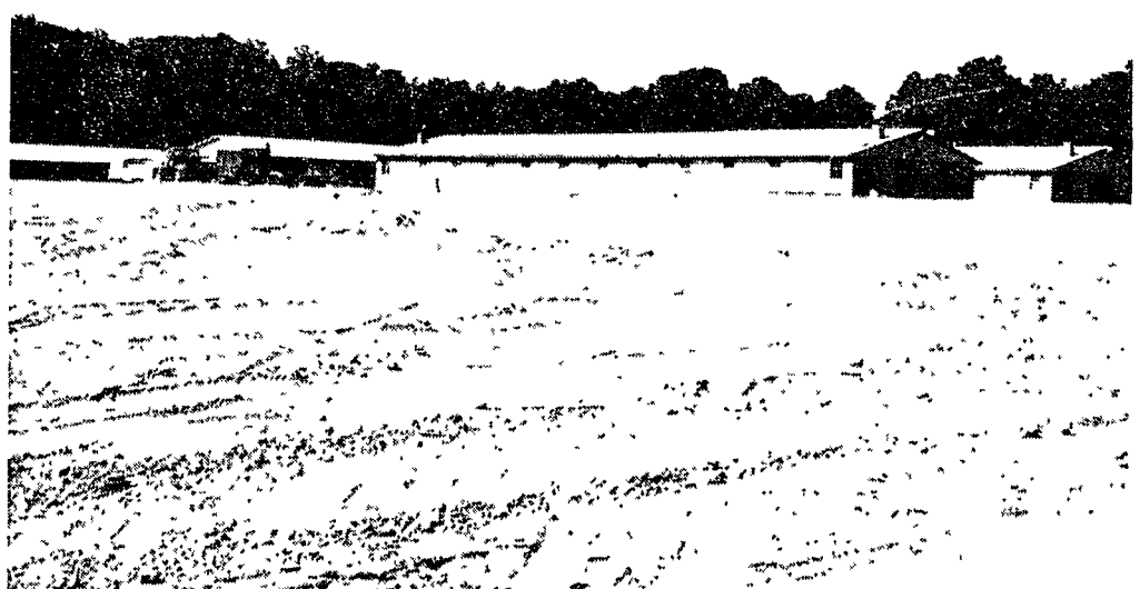
Bulldozers pushed some 50,000 yards of earth to make this new area next to the Sheldon road barns this spring. In about two years, when earth has settled, seven more barns will be built.
