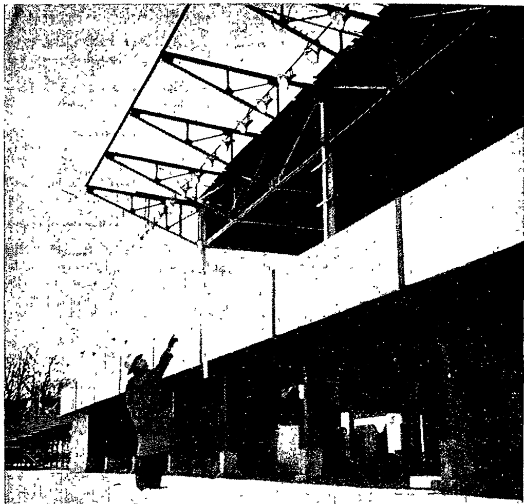
POINTING to the spot in the grandstands where the new judges' stand will be located is Downs' Executive Manager John Carlo. Revamping of the stands is already underway, as evidenced by the improvements made in the box seat area in the foreground. New beams support the section, while pre-cast concrete slabs extend the full length of the stands in front of the box seats. The judges stand will be suspended from the roof section, shown partly dismantled. Carlo expects to spend $75,000 to improve the stands this year. His long-range program calls for further improvements to the stands and construction of a clubhouse where the bleachers now stand. Total estimated cost of this would be $1½ million.
