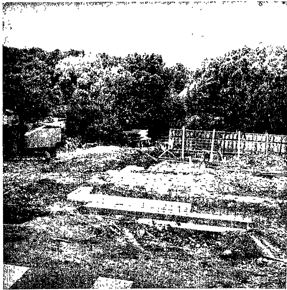
CONSTRUCTION of Northville's new Kroger supermarket was underway full scale this week. Footings have been poured, houses in the area will soon be removed. Early fall opening of the 16,000 square foot store is planned.
