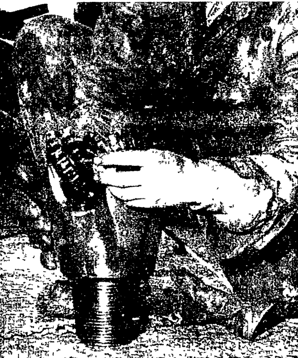
DRILLING BIT — Drilling through iron-hard rock requires a bit of special alloy. Even so, bits wear out and must be replaced. Here workmen look over one of the worn out bits used at an exploratory well in Salem township.
