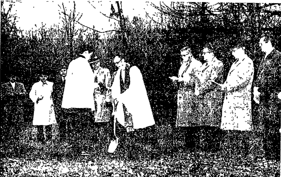
NEW CHURCH — The Reverend John W. Miller turns the first spade of earth at groundbreaking ceremonies Sunday for a new church of the Evangelical Lutheran Church of the Epiphany will build on a six-acre site on Five Mile between Bradner and Haggerty roads in Northville township. Present plans call for construction of one unit consisting of a wing for worship and a second wing to house a fellowship hall, classrooms and an office. It will encompass about 5,000 square feet. Completion is expected within 180 days. About 65 members of the church, a mission of the United Lutheran Church of America, traveled to the site Sunday from their present place of worship in Plymouth. Representatives of the building committee and church council who took part in the ceremonies were: Gilbert Pearson, Steve Seregan, Fred Meier, Cecil Ronk, Harlan Hickerson, James Anderson, Charles Johnson and Clarence Iverson. Robert Robinson, assistant to the president of the Michigan synod, also attended along with James Morison, architect of the structure.
