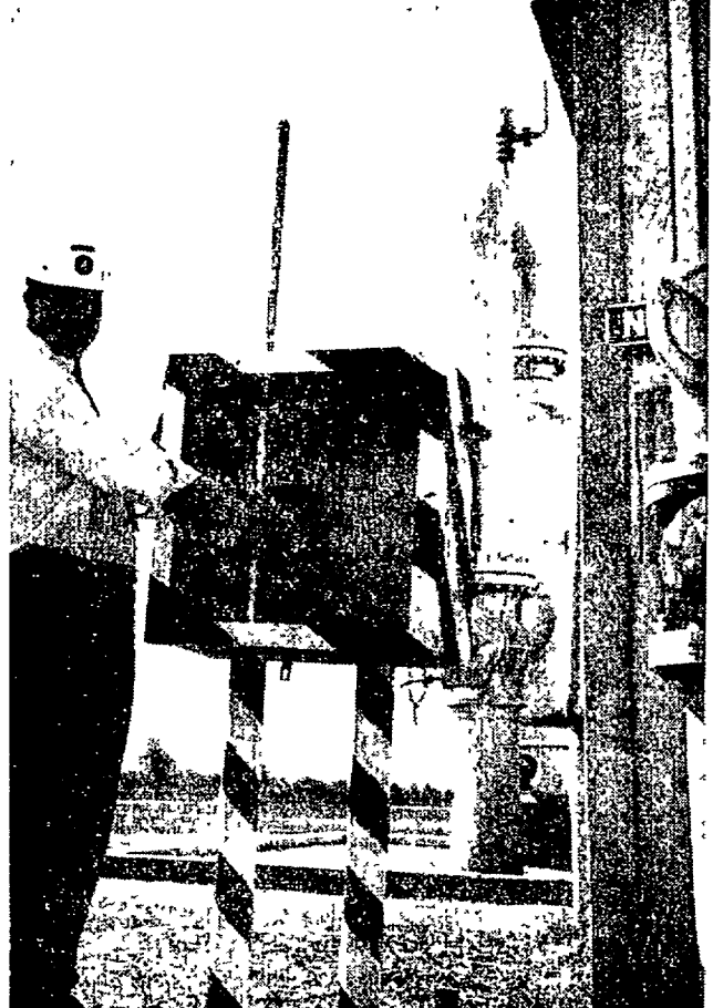
SAFETY FIRST — A twist of the wrist and Floyd Neff, pumping station superintendent, could shut down Consumers Power company's Northville station. The valve he's holding closes off incoming and outgoing pipe lines, shuts down the giant engines and compressors, disconnects the main power line and emergency generator and opens a blow-out valve to clear all pipes in the station. All operations except the blow-out require only 15 seconds. The blow-out would be completed within four to five minutes. Consumers has five such emergency stations located in its pumping facility. They would be used in case of a ruptured live, fire or other danger that could cause an explosion.
