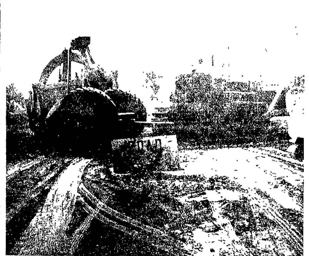
WEST ROAD in Wixom receives "the big move" treatment from huge earth movers and bulldozers. The contractors discovered large deposits of muck under the road bed, which had to be dug out and replaced with solid dirt before the new road bed could be constructed. The contractors are scheduled to finish off the south end of Beck road and rebuild Loon Lake road this summer in the city's $80,000 road building program. Paving of all three roads will be done later.
