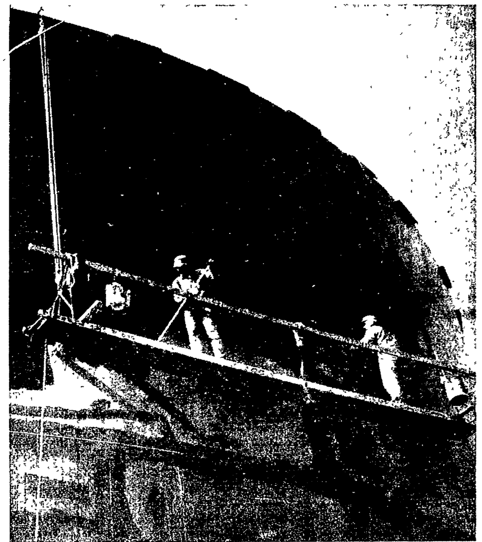
Two painters — Dale Bonnell and Carl Maier — swab the storage tanks with a coat of rust-proof. They'll get a coat of white later.
