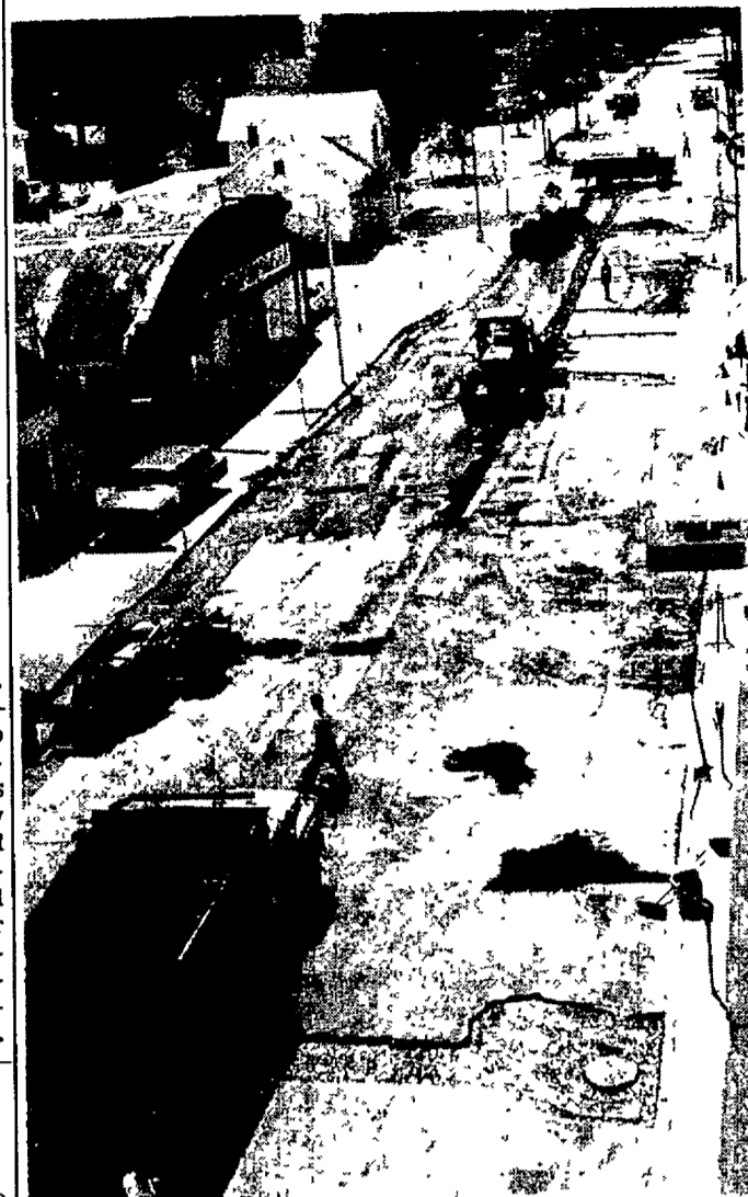
BIRDEYE VIEW—This aerial shot of Main street shows repair crews at work removing deteriorated areas and preparing the street for repaving. Main street from Rogers to Hutton will receive a one-inch asphalt overlay when the patch-work is completed. Paving on Dunlap from Rogers to Center was completed Monday. The Dunlap improvement will be continued to Hutton. Paving on Main street from Rogers to Wing is planned for completion this week. Paving to Hutton will be completed after the holidays. Thayer, Cady and Eaton drive are then in line for resurfacing. The entire job is scheduled for completion by mid-July.
