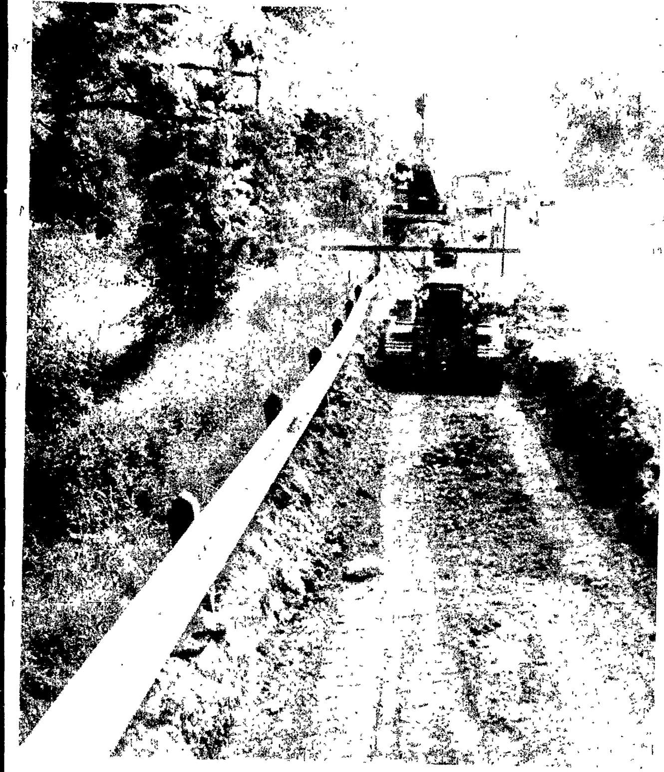
FIVE MILE BOUND —Contractors extending the Detroit water line from Baseline road in the city of Northville to Five Mile and Sheldon road were approaching Six Mile road this week. When the installation is complete to Five Mile, the crews will return to the city and connect the line from Fairbrook at Center (Sheldon) to a point just south of Seven Mile road on Sheldon. The work from Fairbrook south was discontinued when the races started at Northville Downs June 21. It cannot be resumed until after the summer meet closes August 4.
