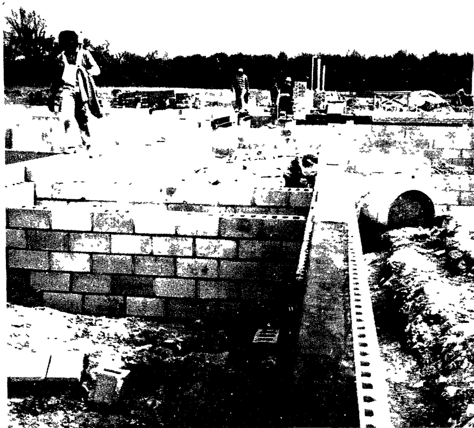
KNEE HIGH SCHOOL —Northville's new elementary school on West Eight Mile road reached the knee-high level this week as work resumed after a brick and block-layers' strike curtailed activity at the site for nearly two weeks. E.V. Ellison, director of administrative services for the school system, said Tuesday that a September opening of the 17-room facility is still planned, although the project is admittedly behind schedule.
