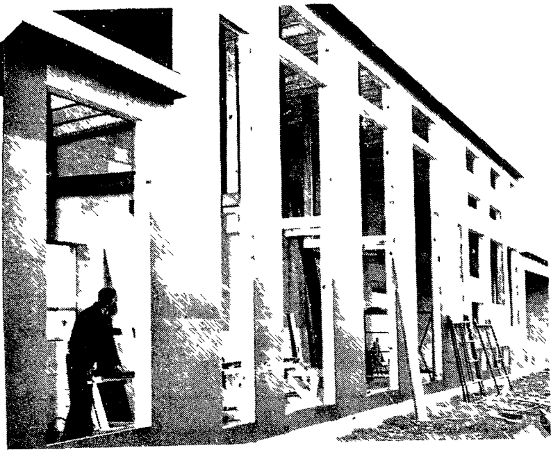
NEW TOTE BOARD —Construction of a giant new tote board is fast nearing completion at Northville Downs. The 100 x 20-foot board, required under state racing laws for tracks that show an average daily handle of $250,000 for three consecutive years, is situated near the center of the track infield. Besides flashing racing odds, the new board will
