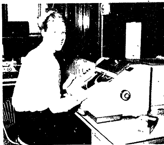
Headlines are her specialty. Merle Duey sets them on the Varityper Headliner.
