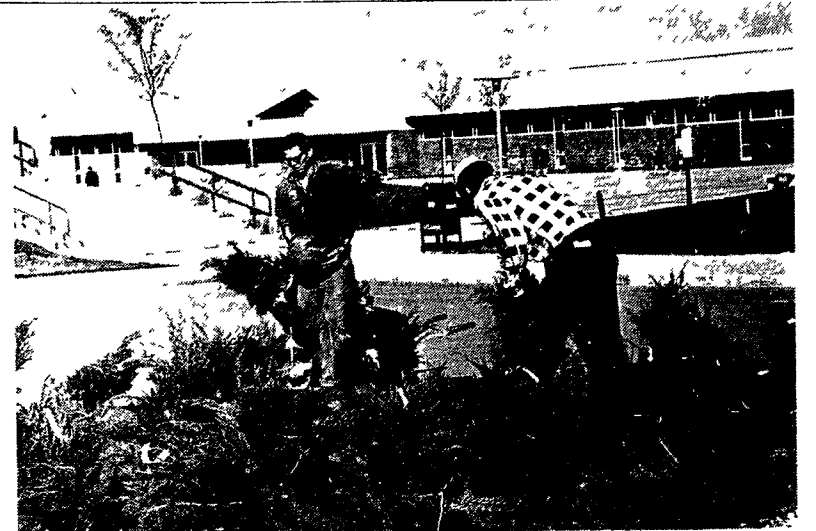
CAMPUS LANDSCAPING —Workmen set one group of the nearly 200 low spreading junipers to be planted as part of a major landscaping program underway at the 139 acre Schoolcraft College campus. This first phase of the
