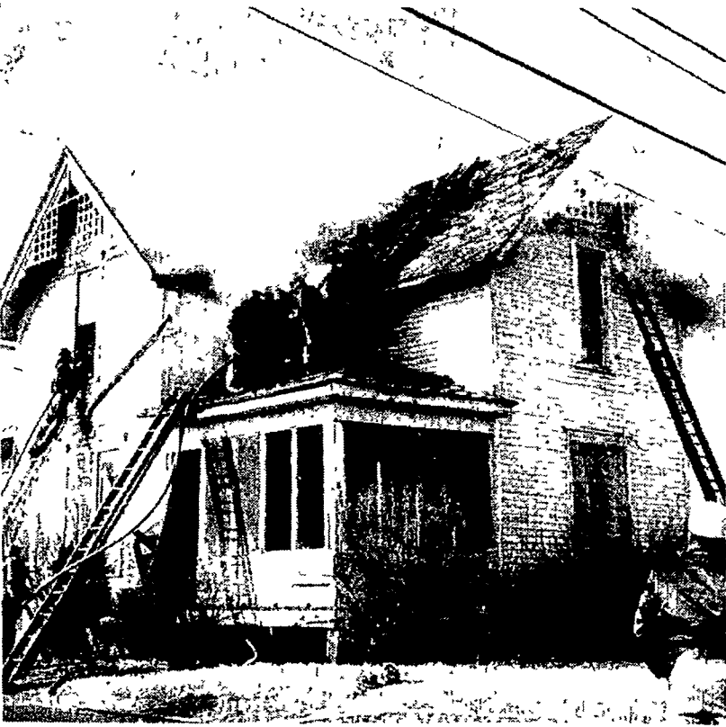
HOUSE GUTTED - Still tasting smoke from a series of grass fires this past week, Northville firemen joined the Salem department Tuesday morning in battling a blaze that gutted a 10-room frame farmhouse at 53853 West Eight
