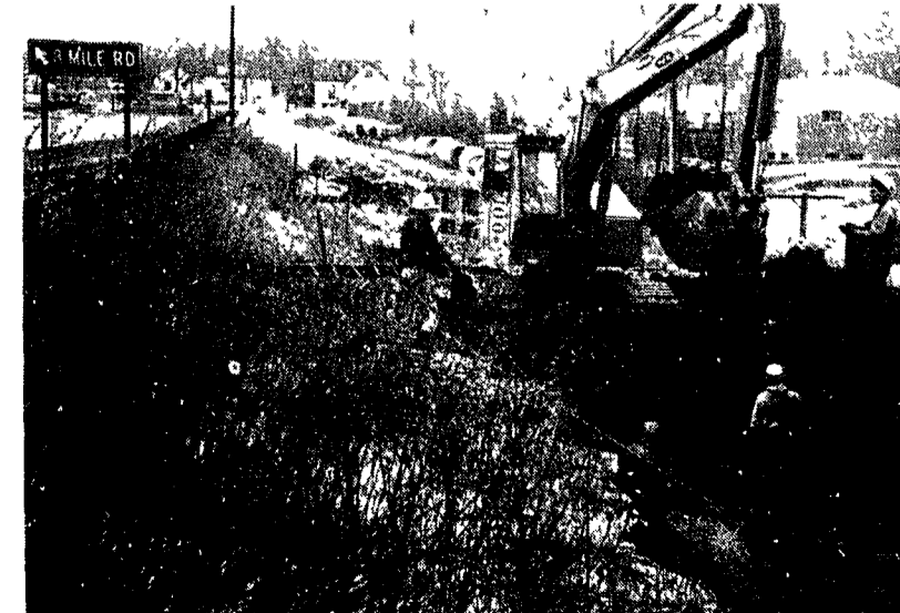
STORM SEWER—Construction of the new Maplewood-Nowi storm sewer, costing $73,546, got underway this week as workmen began laying the 42-inch tile along the Eight Mile Road cutoff between Novi Street and Novi Road.
