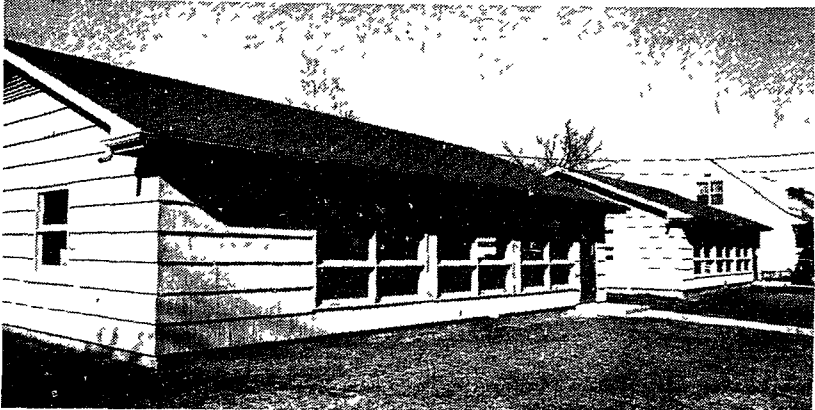
THE CUMMINGS ELEMENTARY Units from the exterior still blend into the neighborhood. In the South-western section of Flint, they were among the first of the 140 units now in operation. Constructed in 1954, the first grade and kindergarten units pictured show how one general pattern of architecture was followed to effect the $10,991 cost per unit.
