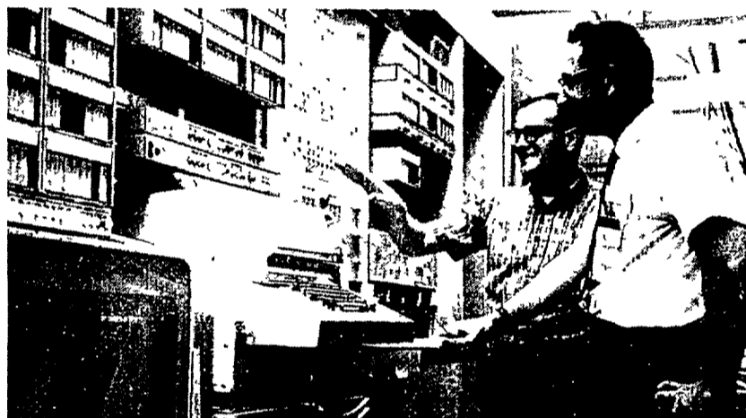
SWITCHMAN Robert M. Hutchens (left) and chief switchman Joseph B. Congiolo test the huge new long distance switching machine housed in a three story building in Plymouth. Teletype unit at left helps pinpoint a component failure and is used to give new orders to a vast array of switching equipment.
