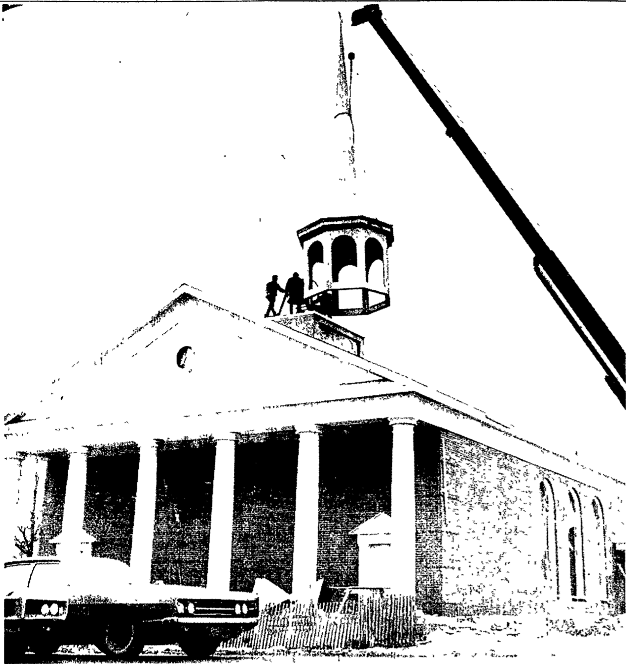
STEEPLE GOES UP - Trucked in from Georgia Thursday, the steel and fiberglass steeple belfry for the First Presbyterian Church of Northville was assembled on the ground and then hoisted to the roof of the new sanctuary where it houses the church's historic old bell.
