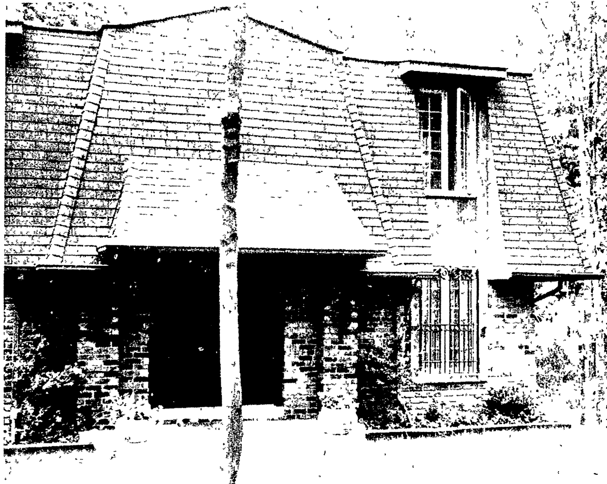
NESTLED DEEP IN WOODED SETTING, HOME FEATURES MANSARD ROOF
