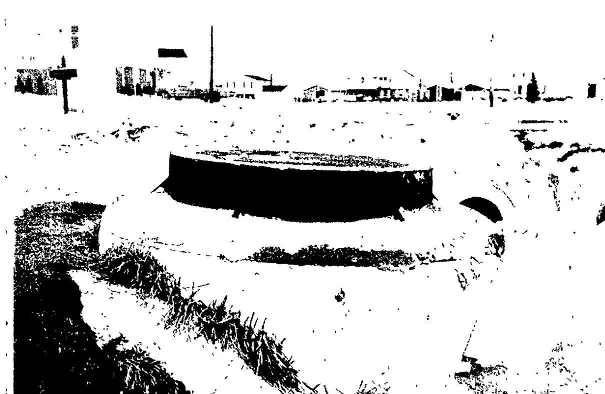
...AND PROTRUDING SEWER RISERS GRIEVE CITIZENS IN MEADOWBROOK LAKES.
