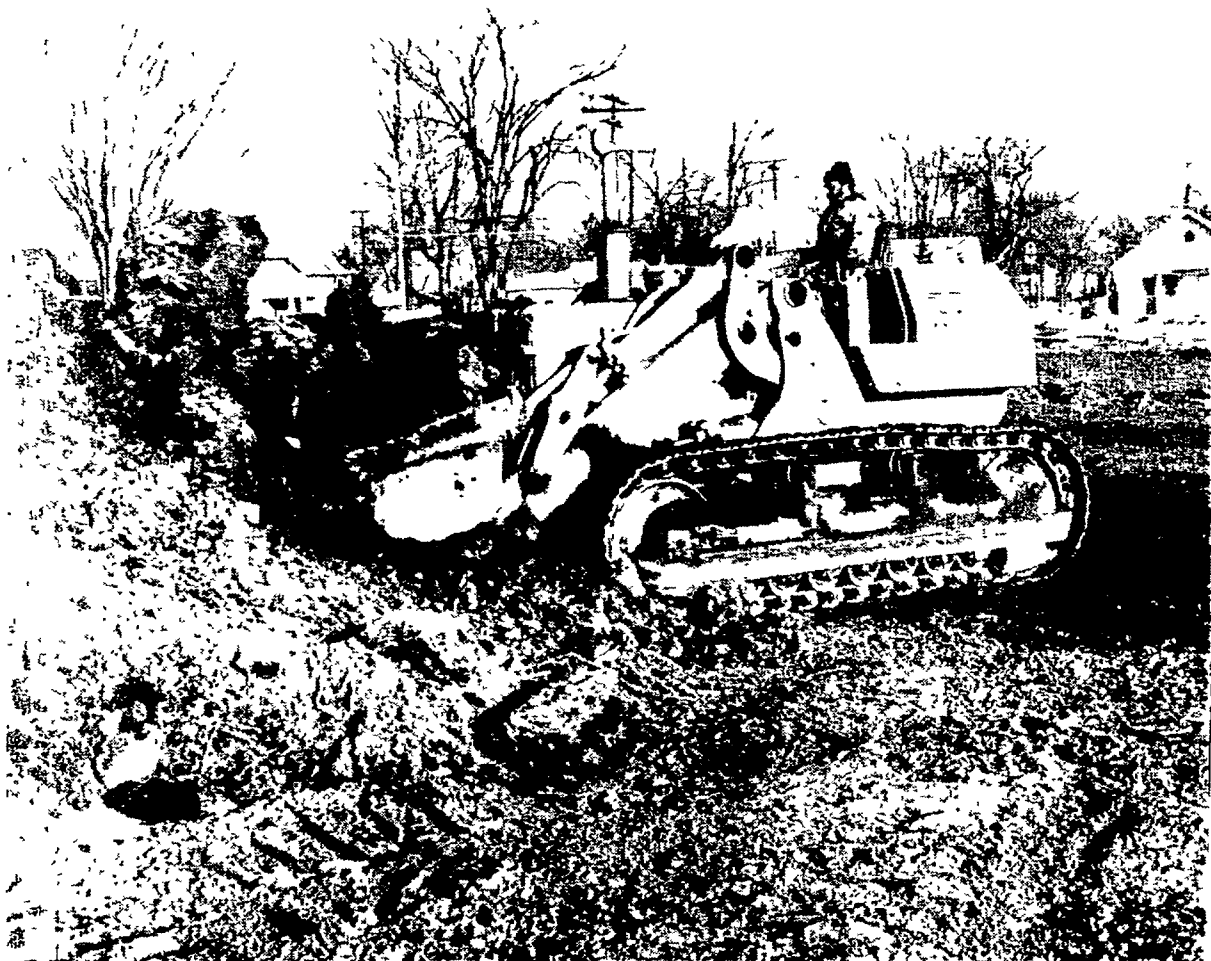
DIGGING UP A SUPERMARKET — Hungry earthmovers began eating into the site for the new Chatham supermarket, to be located on North Center Street, early last week. Foundation construction is expected to begin soon, and Chatham officials remain hopeful that the new facility will be completed for opening later this year.
