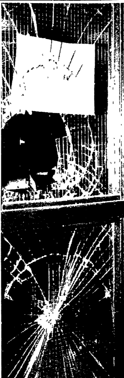
SHATTERED — Vandals rammed this window with a fire extinguisher during a spree of destruction Sunday night at Cooke Junior High.
