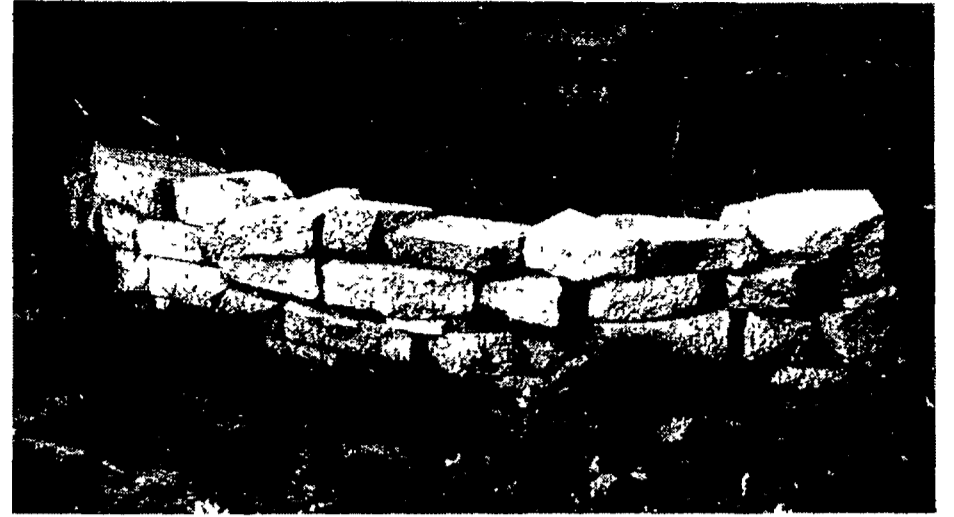
A WALL of uncemented stones or blocks does a good job of holding and concealing a compost pile. Structures should be located where they are easy to get to but not conspicuous. This one is located in an out-of-the-way corner along a backyard fence.
