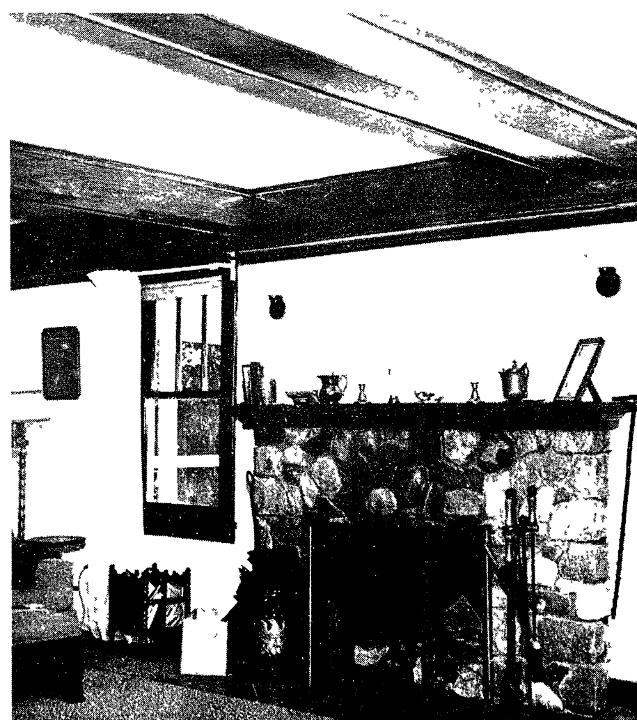
ORIGINAL — The Charles Ware home, 50770 West Pontiac Trail still sports the original 14" hand-hewn beams with which it was built 160 years ago. No nails here either, beams are held together by wooden pegs.
