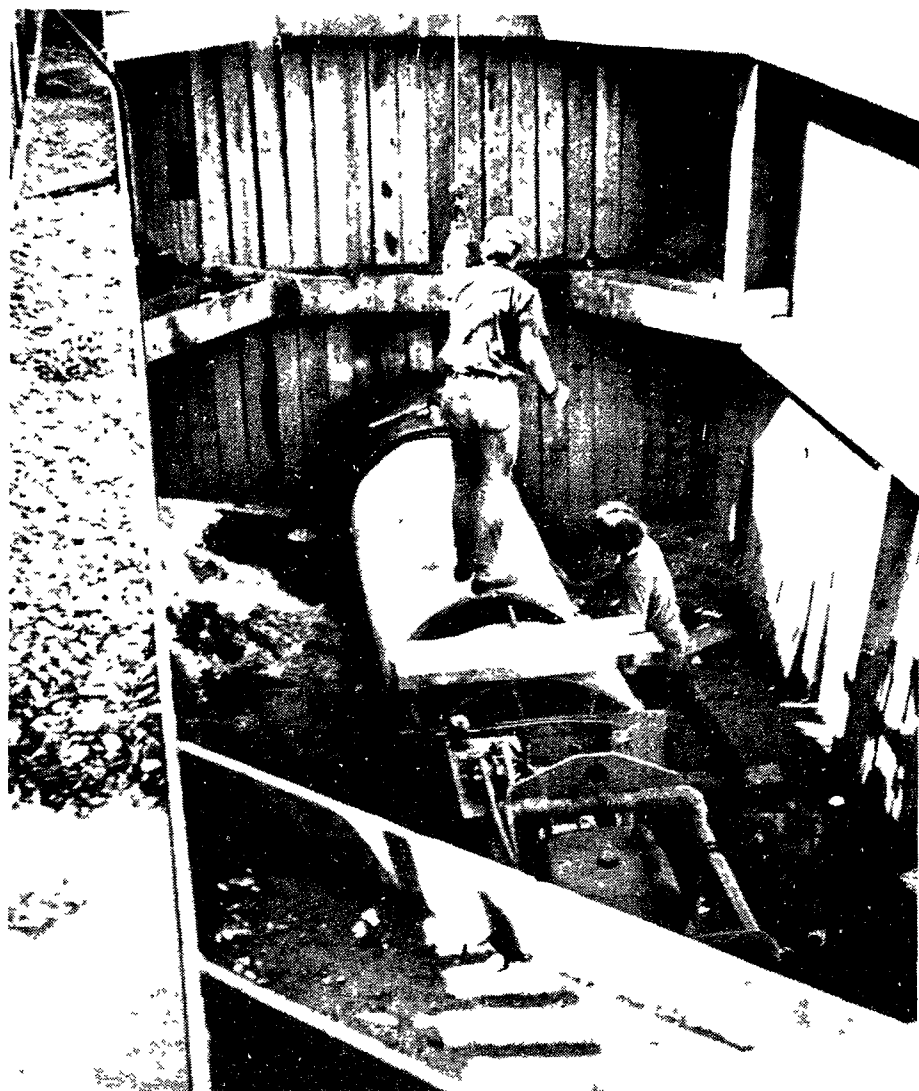
NEARING COMPLETION — Workmen are busy completing the final hook-up that will make the 11 Mile sewer-arm operable and enable the Middle School to hold classes. Shown here tunneling beneath the railroad tracks on 10 Mile Road, workmen must finish this tie-in with the major line before the 11 Mile extension can be used.
