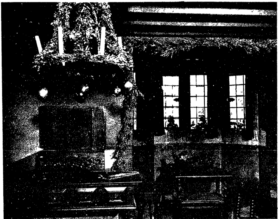
EARLIEST DECORATIONS —The Cotswold Cottage from England, which dates back to 1620 and is the oldest house in Greenfield Village, is decorated for the holidays with a "kissing bell" of boxwood, cedar garlands, holly, candles and apples. All decorations in homes open in the village are authentic to the period of the house. They are open through January 2, excepting Christmas and New Year's Day.
